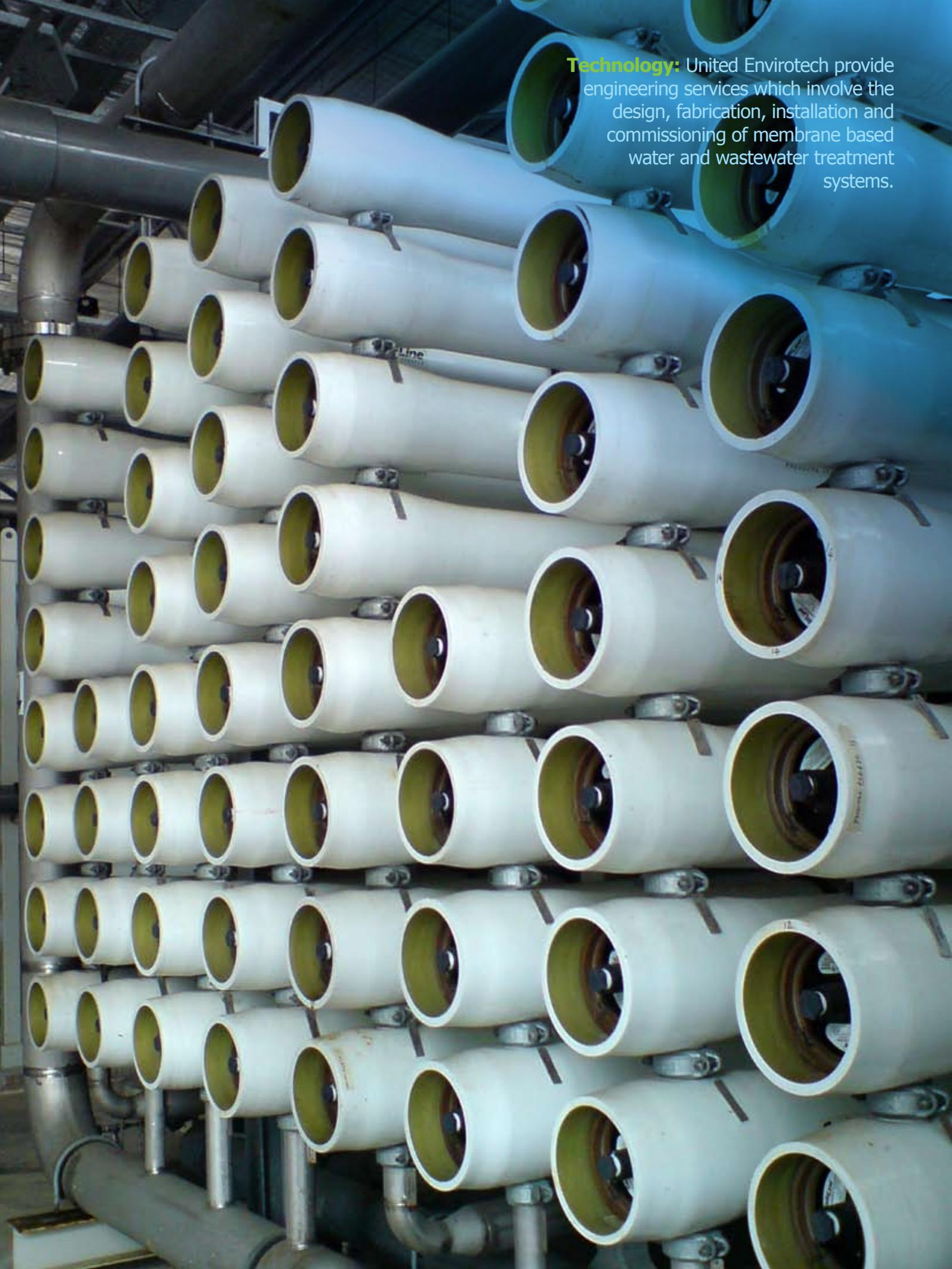
The image shows a dense array of white, cylindrical membrane modules arranged in multiple rows. Each module has a circular opening at the end, revealing internal components. The modules are connected to a network of grey pipes and metal fittings. The overall scene is an industrial setting, likely a water treatment plant. In the top right corner, there is a text overlay in white and yellow.
